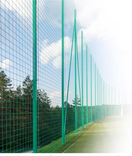
Fixing the net in the lower and upper part to a 3 mm thick steel wire rope using galvanized steel snap hooks.
