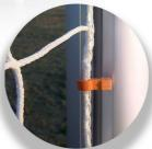
The net is attached to the goal frame and bottom frame with PP hooks.
