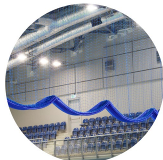
Curtain during lifting, lowering.
